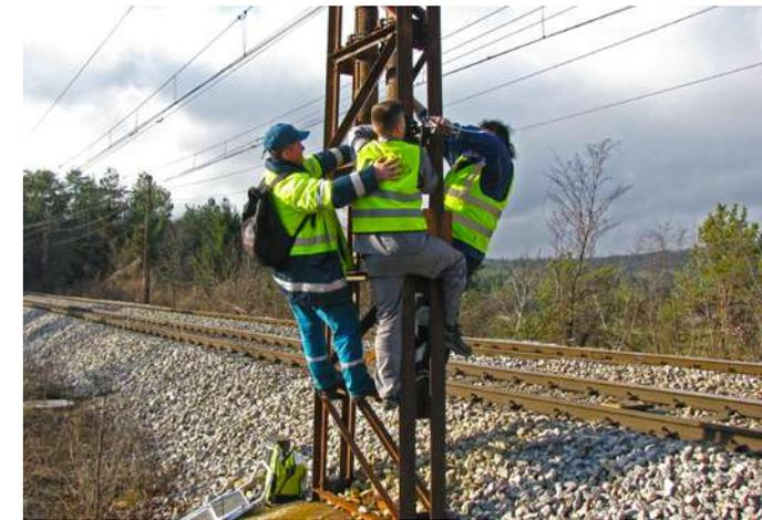
Installation of acoustic deterrents on electric poles along railway section.
