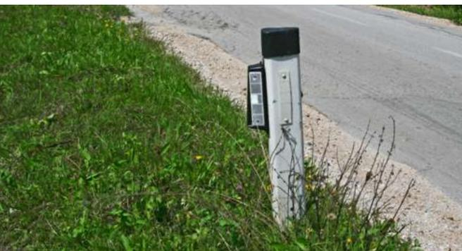
Acoustic deterrents are placed directly into roadside pillars.
