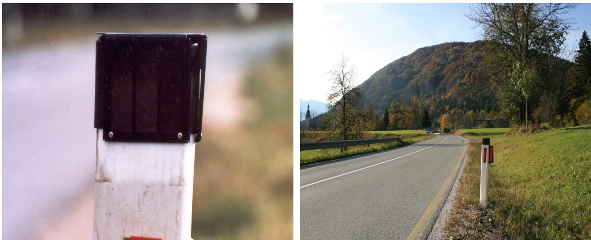
Figure 2: Two types of acoustic deterrent that have been used so far in Slovenia.
