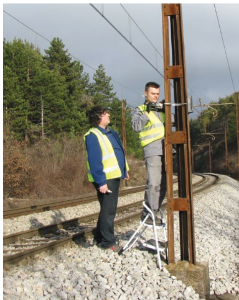
Acoustic deterrents were installed on electric poles along the railway tracks in Slovenia to reduce train-bear collisions.
