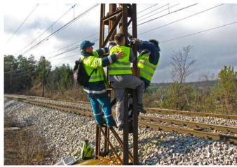
Installation of acoustic deterrents on electric poles along railway section.
