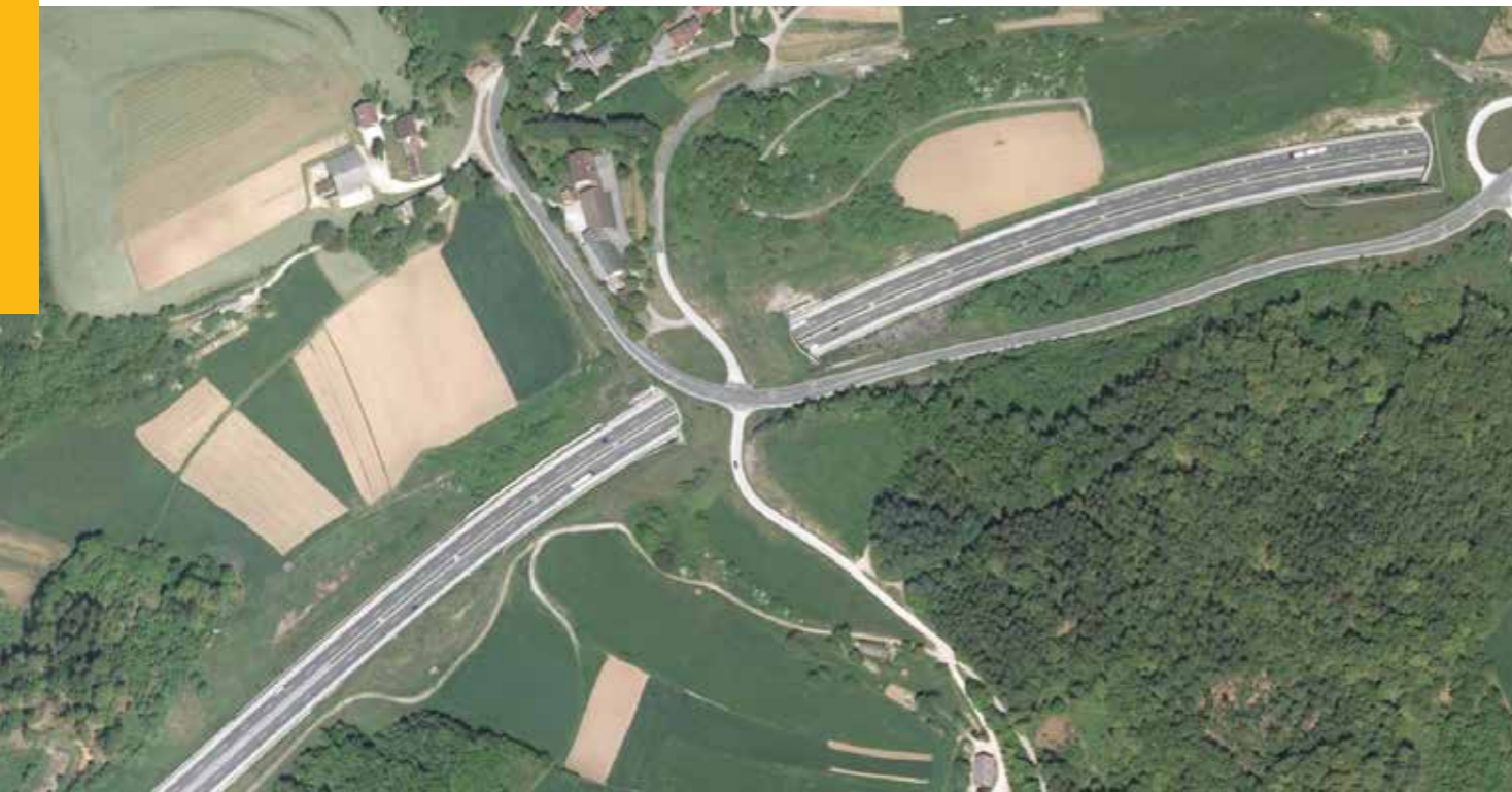
Example of multi-use overpass at Veliki Gaber (motorway Ljubljana – Zagreb), where local roads and dirt roads have been built over the pass. After the construction new housing infrastructure has been built which additionally decreased the suitability of the overpass for large mammals. (Atlas okolja)
