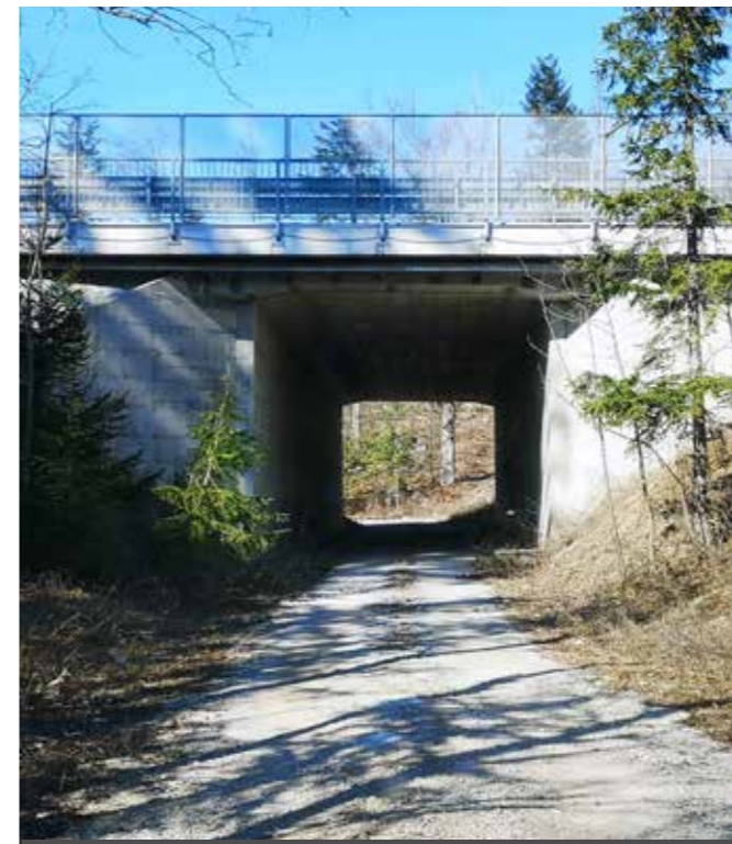
In addition to the location, the permeability of underpasses for large mammals also depends on the width, height and length of the structure, defined as openness index. Left: A lower openness index is unsuitable for the passage of certain types of large mammals. (Črtalič J.) Right: Underpass, under which a stream flows, is located on the edge of the underpass. (Potočnik H.)
