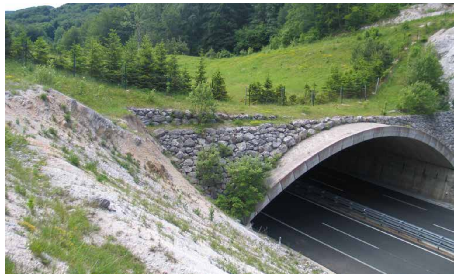
Adequately placed green bridges are the most effective crossing structures to mitigate fragmentation effects in large mammal habitats, especially for large carnivores. (Huber Đ.)
