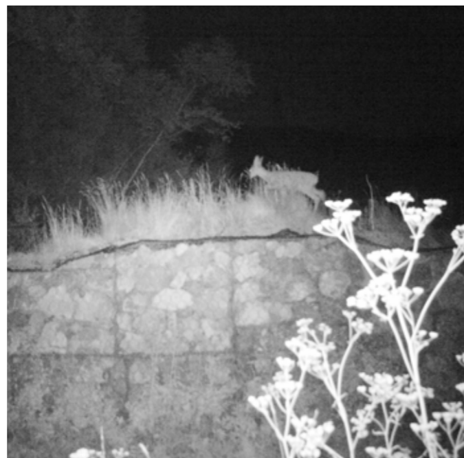
Monitoring the effectiveness of jump-out ramp that allows animals that do manage to get onto fenced motorway Zagreb - Rijeka, to quickly leave the area. (Huber Đ.)
