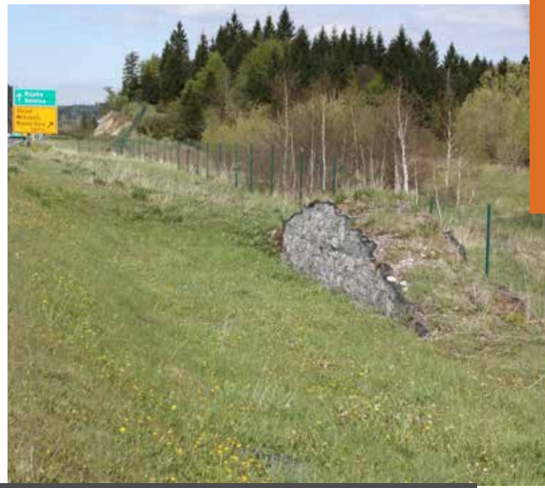
Escape exit doors and jump-out ramps are used to allow animals that have managed to get onto fenced motorways a quick and safe exit from dangerous area. (Huber Đ.)
