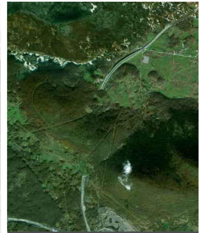
Area above the tunnel remains completely preserved which is especially important when it has an important ecological role, like connecting habitat patches. (tunnel Plasina, CRO)
