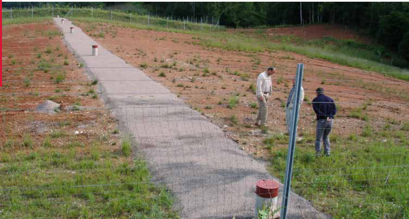
Sand beds on green bridges are often combined with animal counters, which allow the evaluation of the frequency of the passage of individual animal species, based on footprints that are recorded in the sand. (Huber Đ.)
