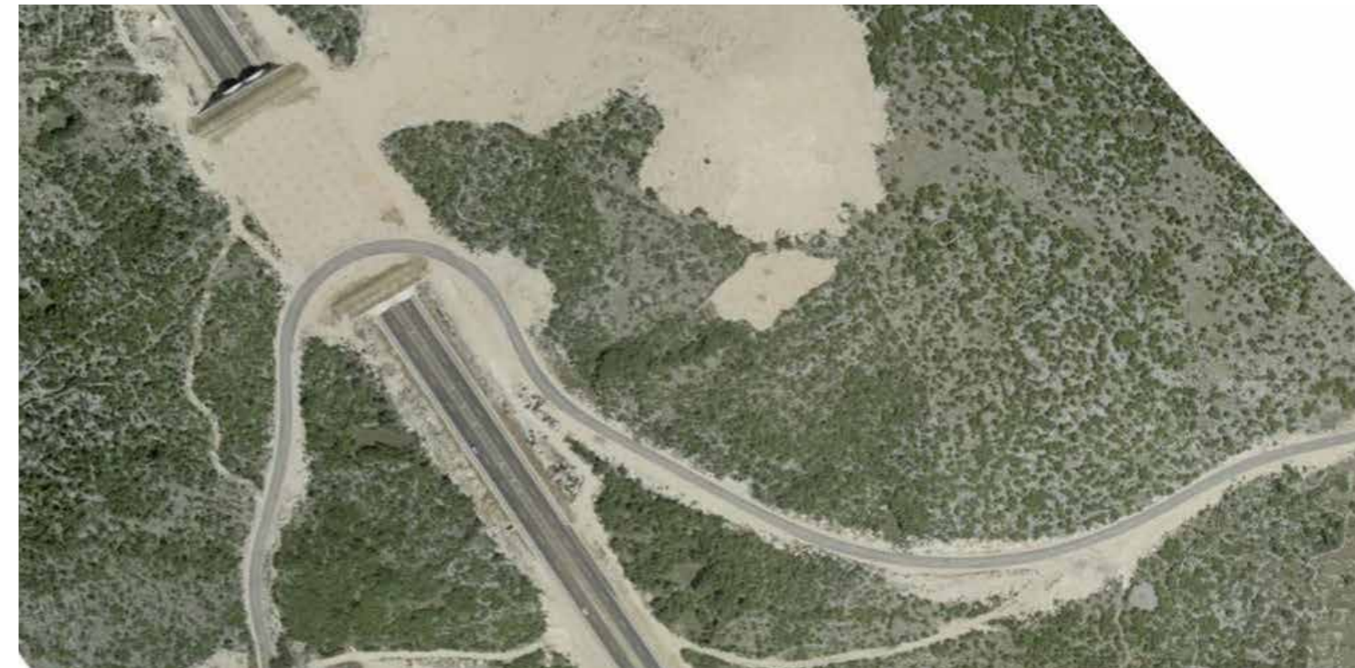
Example of inappropriate construction of green bridge (Vranovića ograda, Croatia) where local road has been constructed over the bridge to connect village across highway. Separate road overpass should be constructed instead.
