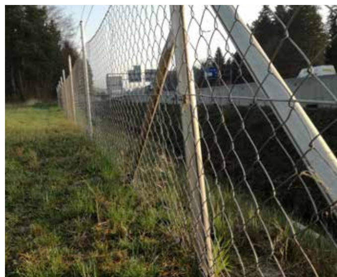
All highways in Slovenia and Croatia are fenced on at least one side with a 160 cm high fence. At some critical section, where bear presence is regular, electrical fences can be added to prevent bears from crossing. (Potočnik H.)
