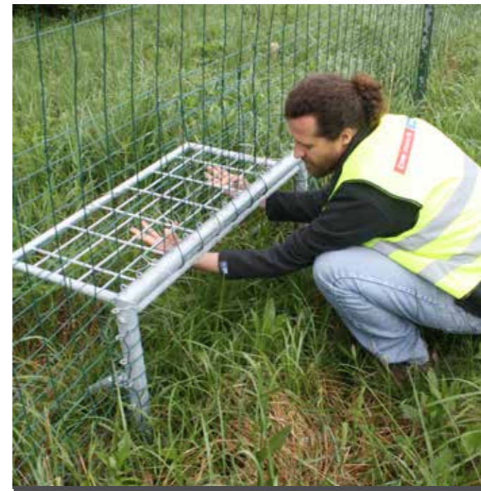
Escape exit doors and jump-out ramps are used to allow animals that have managed to get onto fenced motorways a quick and safe exit from dangerous area. (Huber Đ.)
