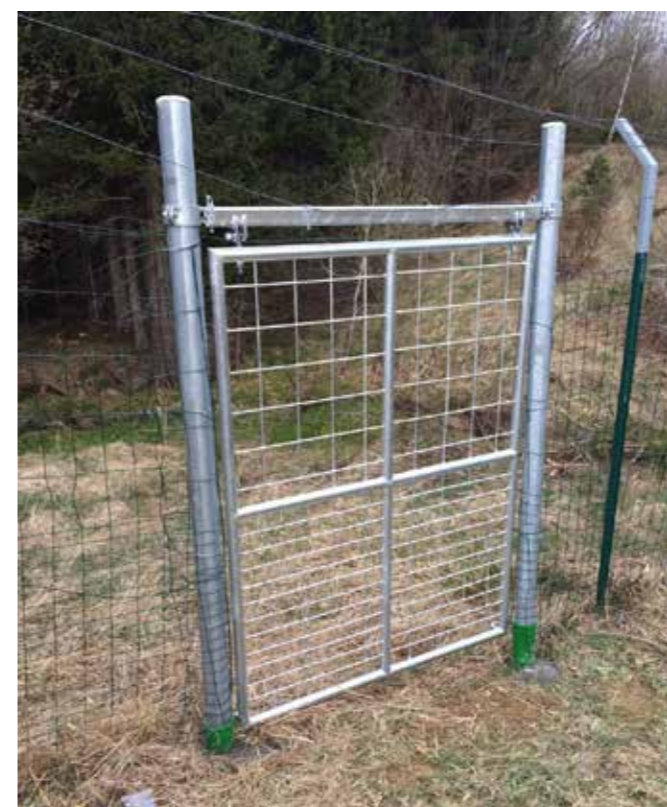
Installation of one way escape doors allows animals to escape from fenced motorway Zagreb - Rijeka (left). Adding electrical fencing ensures protection against bears and guides them to safe crossing locations (right). (Huber Đ.)
