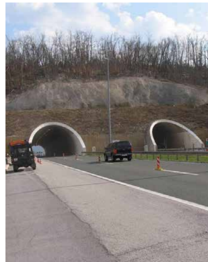
Tunnels provide best solution when planned infrastructure would go through an area of large conservation value. (Huber Đ.)
