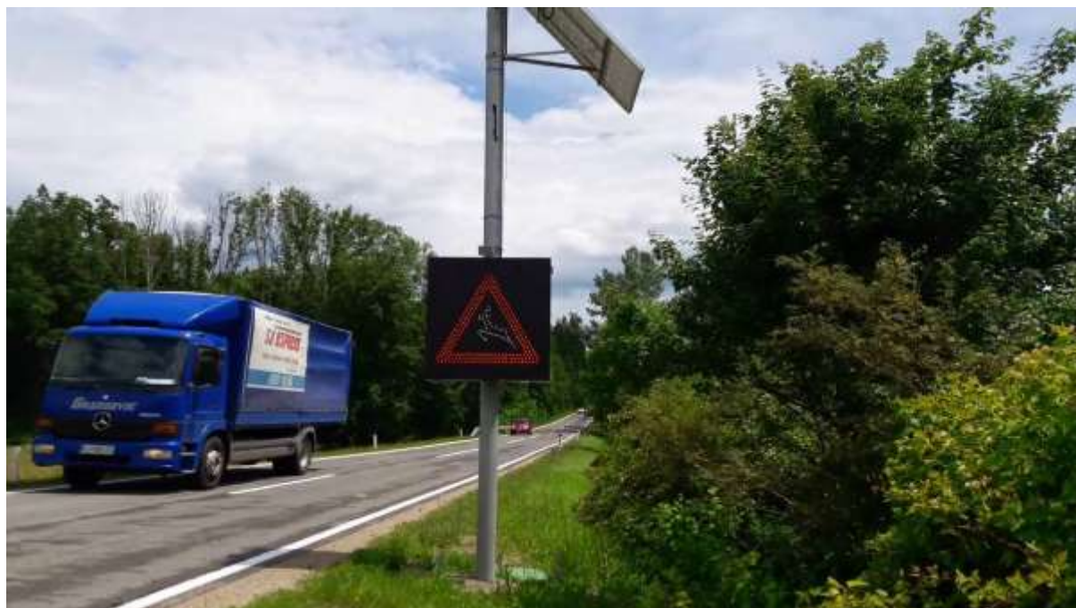
Figure 21: Active dynamic sign at Jasnica (photo: Z. Pavšek, 2016).
