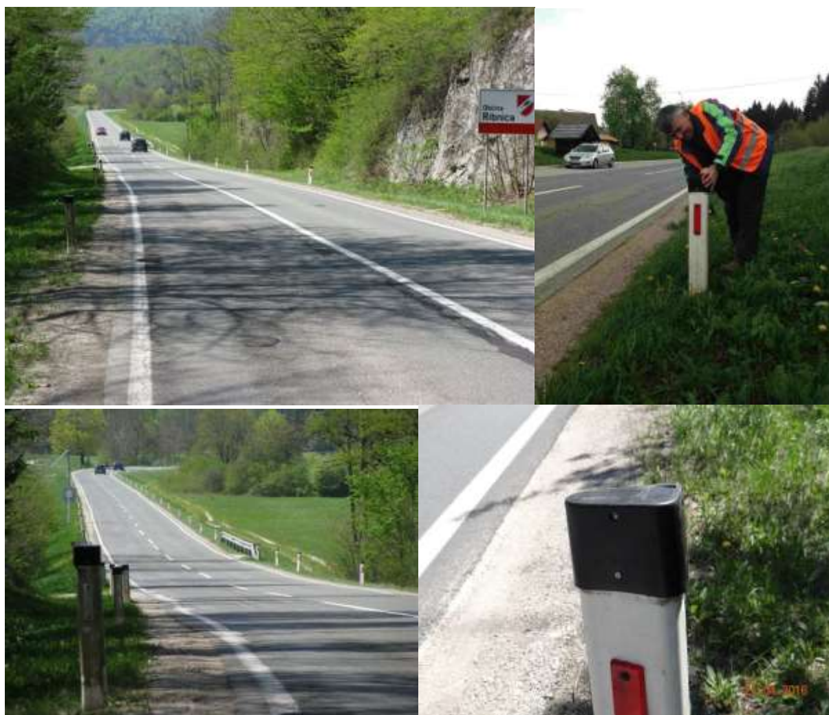
Figure 12: Acoustic deterrents installed along the main road Ljubljana – Kočevje (photo: M. Zaluberšek, 2016).
