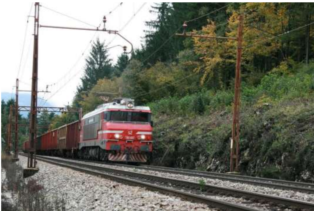
Figure 7: Two types of electric poles to which we installed acoustic deterrents (photo: Z. Pavšek, 2015).
