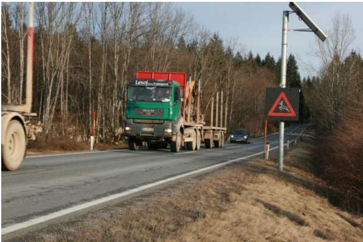
Figure 3: Dynamic traffic signs placed along two sections of the main road Ljubljana – Kočevje (above: Ortnek; below: Jasnica) (photo: Z. Pavšek, 2016).
