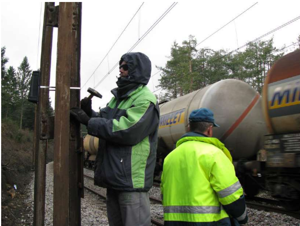
Figure 5: Installation of acoustic deterrents on electric poles along railway sections (photo: M. Zaluberšek, 2015).
