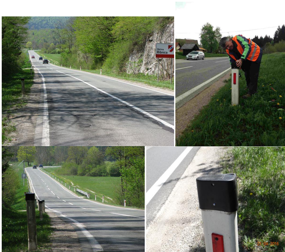
Figure 9: Acoustic deterrents were installed along the main road Ljubljana – Kočevje (photo: M. Zaluberšek, 2016).
