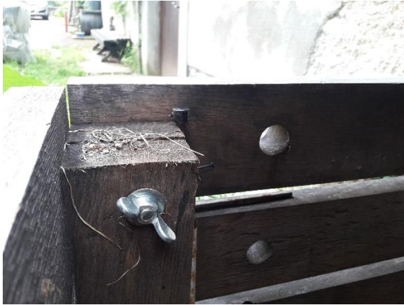
Figure 6: An extra spin added in addition to help open the cover automatically.
