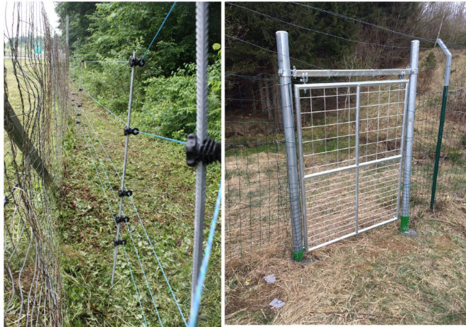
Electric fence along the highway Rijeka - Zagreb. Big one-way exit door on highway Rijeka - Zagreb.
