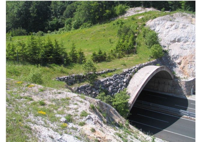
Green bridge Dedin near Delnice constructed for wildlife crossings.
