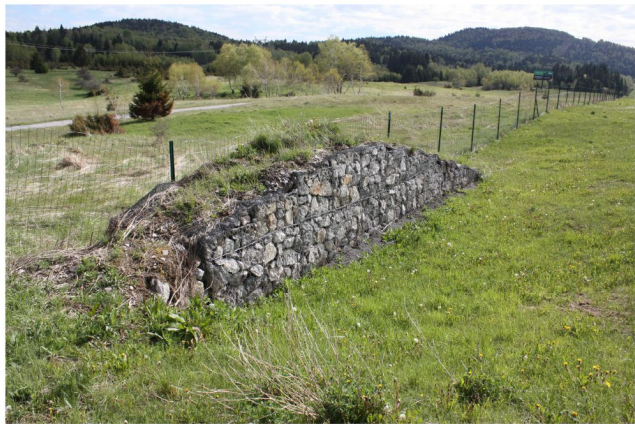
Jump-out ramp for animals to exit the corridor of Rijeka – Zagreb highway.
